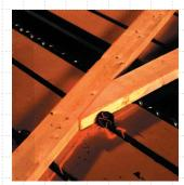
Laser projection showing the "all-up" view which projects on top of thetimber indicating the top plate position.
